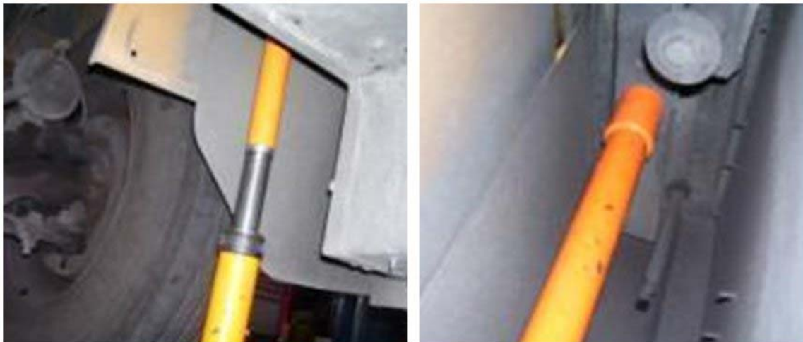
Figure 16 Ram Positioned to Raise RH Side
