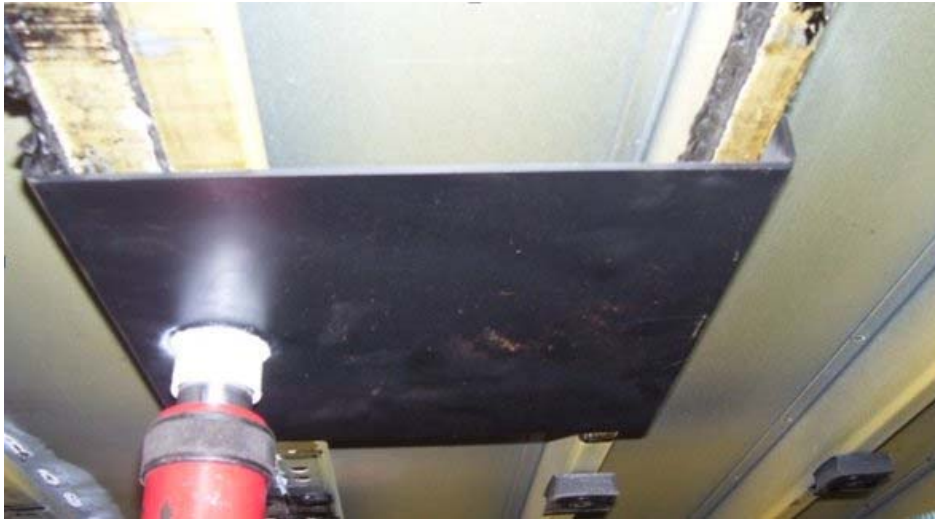
Figure 10 Use a Suitable Plate to Spread the Load Over a Larger Area
